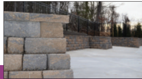
Stone retaining wall surrounding patio area.
