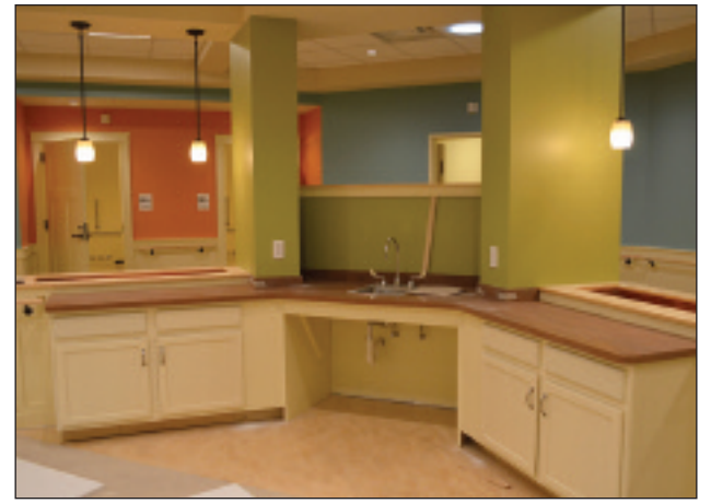
The counter in the arts and crafts area offers plenty of space for clean-up. Along the back of the counter, copper plant boxes will soon be filled with greenery.
